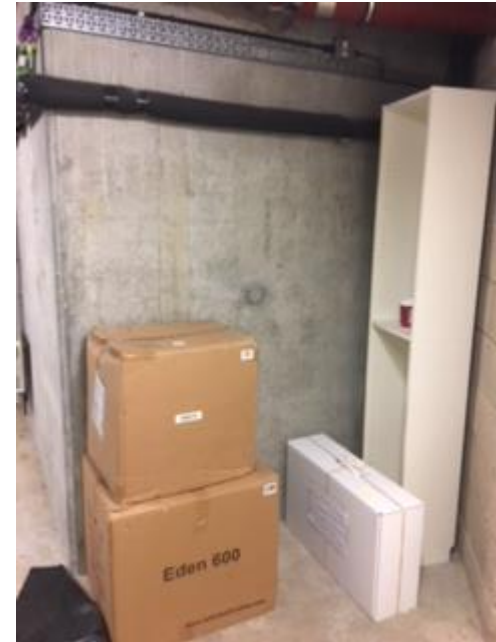
Combustible items within the electrical intake room
