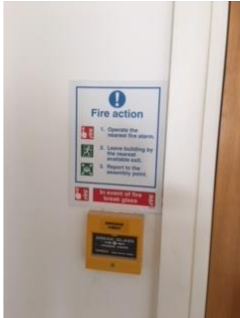
Misleading signage to be removed.
